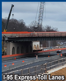
I-95 Express Toll Lanes
