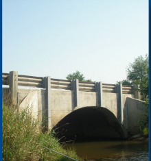
Bridge over Youghiogheny
