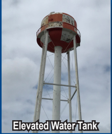
Elevated Water Tank
