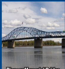
Pioneer Memorial Bridge
